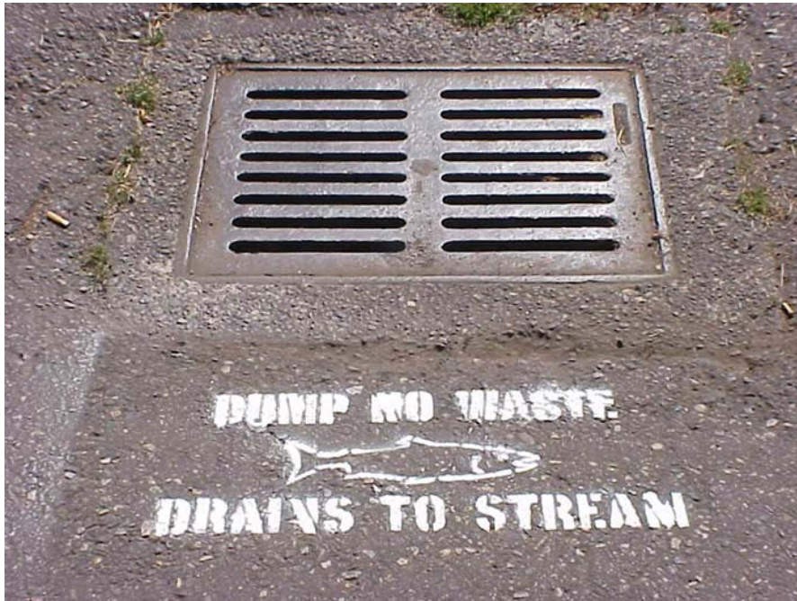
Storm drain that leads to a sewer
