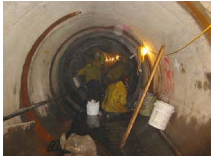
Storm tunnel below St. Paul, MN
